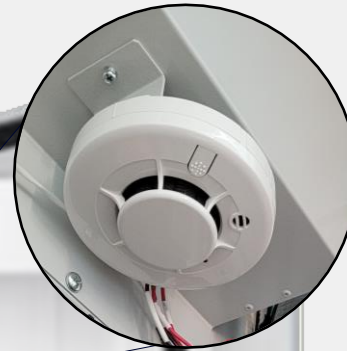
Photoelectric Smoke Detector
